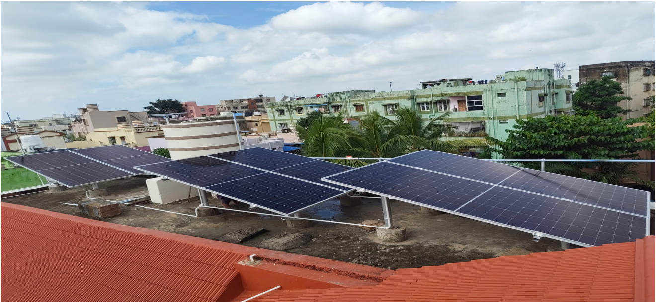
Residential rooftop solar installation • Bhubaneswar, Odisha
